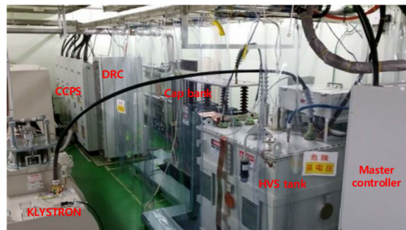
Figure 12: The modulator power supply in iBNCT.
