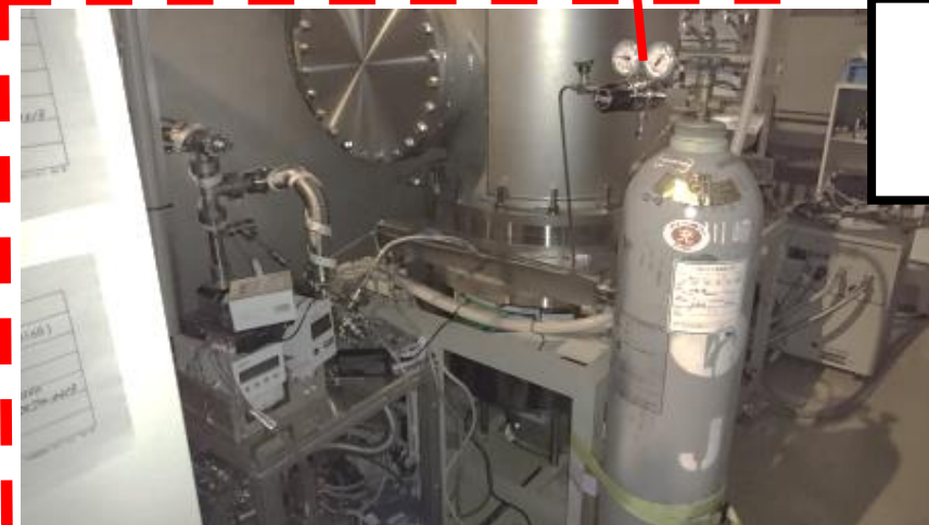
Nitrogen inlet line
