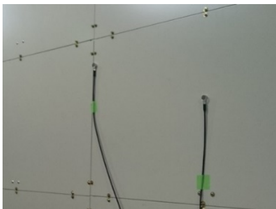
Figure 5: Installation of vibration sensor.
