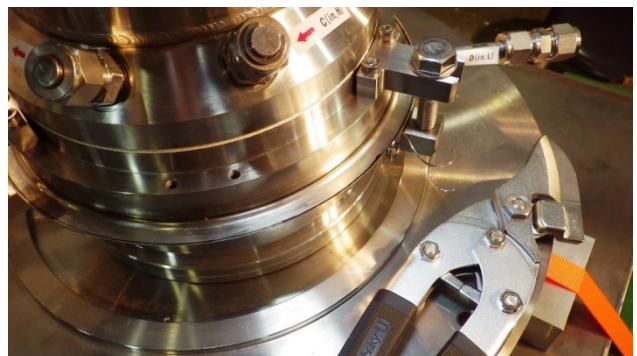
Figure 3: Cutting of the welded lip seal.
