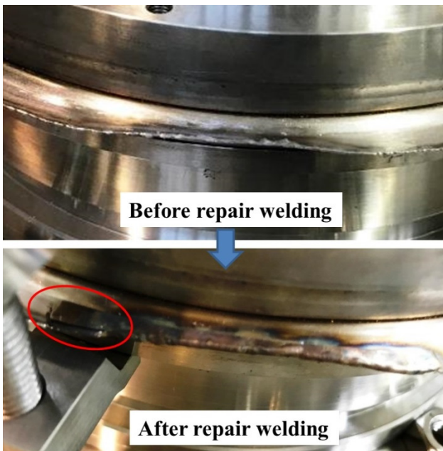
Figure 7: Repair welding where the welding lip is sandwiched by the two stainless steel plates (0.5 mm thick). (Red circle : Leak point after repair welding)
